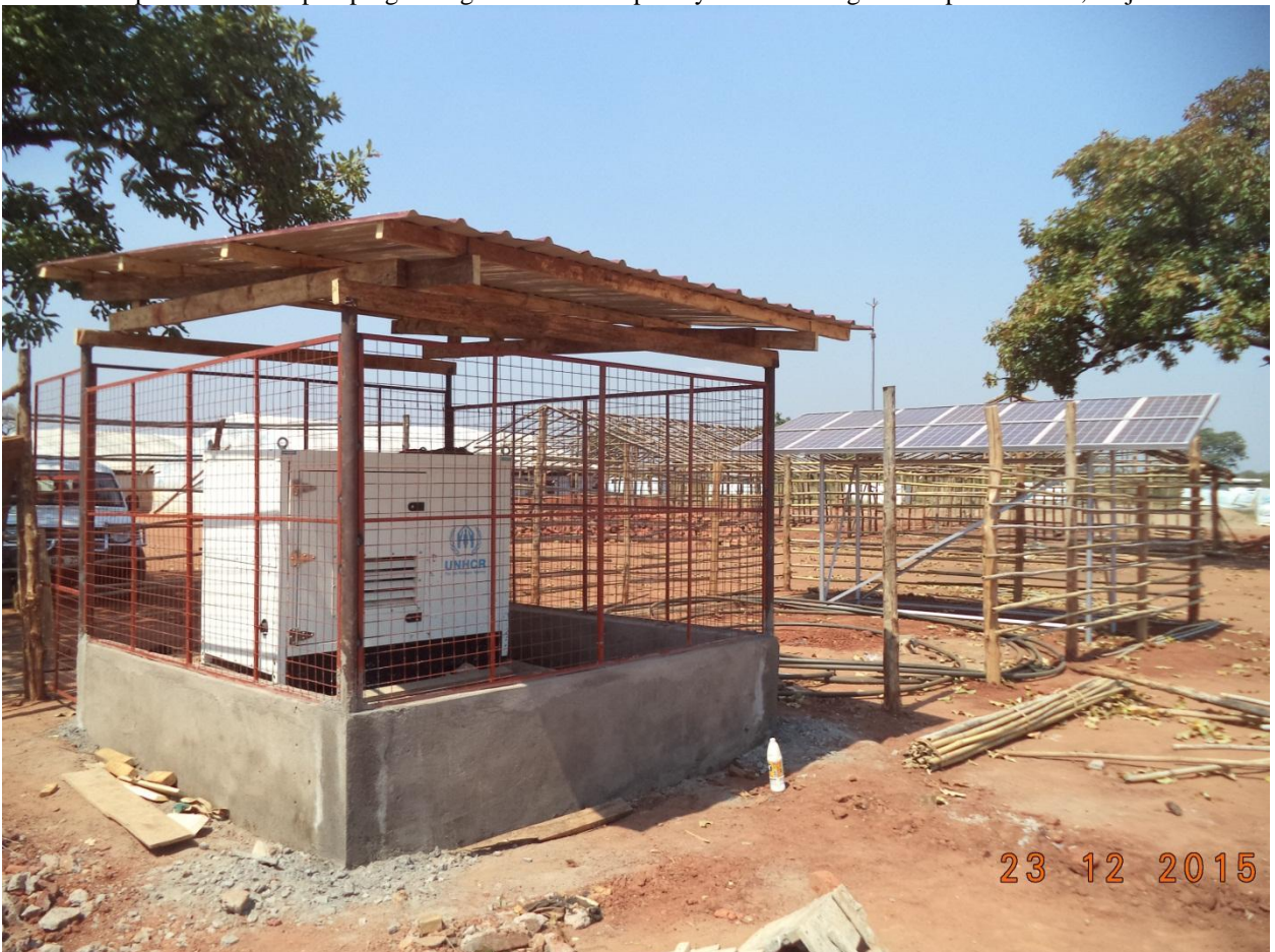
Solar-powered water pumping with generator backup – Nyumanzi Refugee Reception Centre, Adjumani
