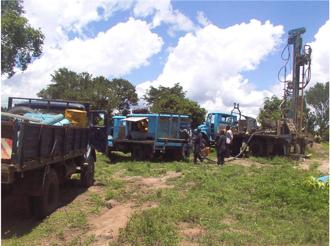
DRILLING UNIT No. 1 – Nabiswa Village, Pallisa District
