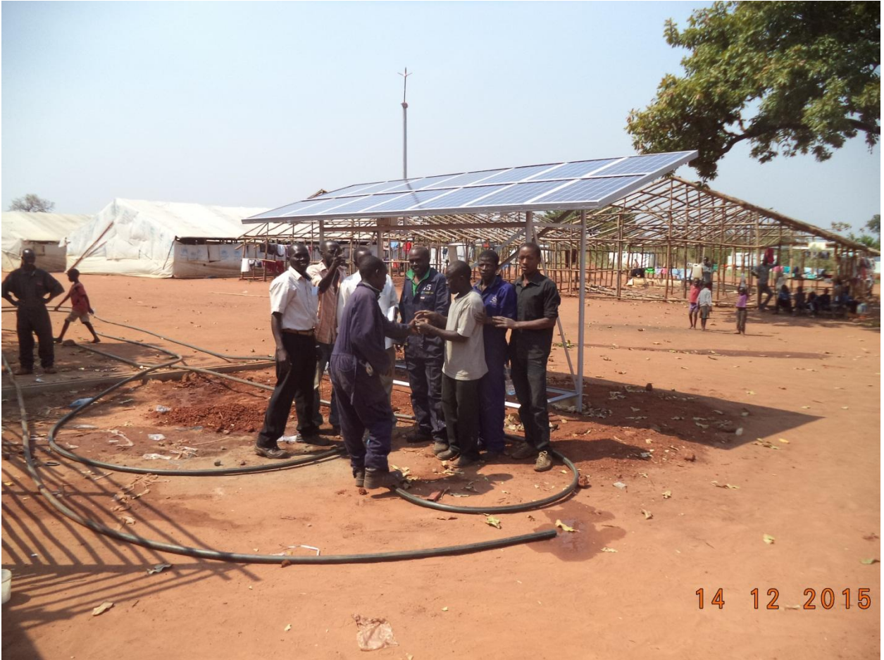
Solar-powered water pumping with generator backup – Nyumanzi Refugee Reception Centre, Adjumani
